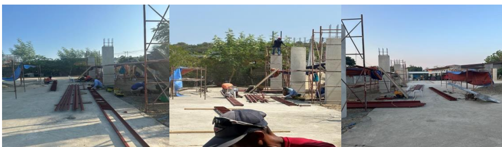
ON GOING PROJECT COVERED COURT BUILDING
