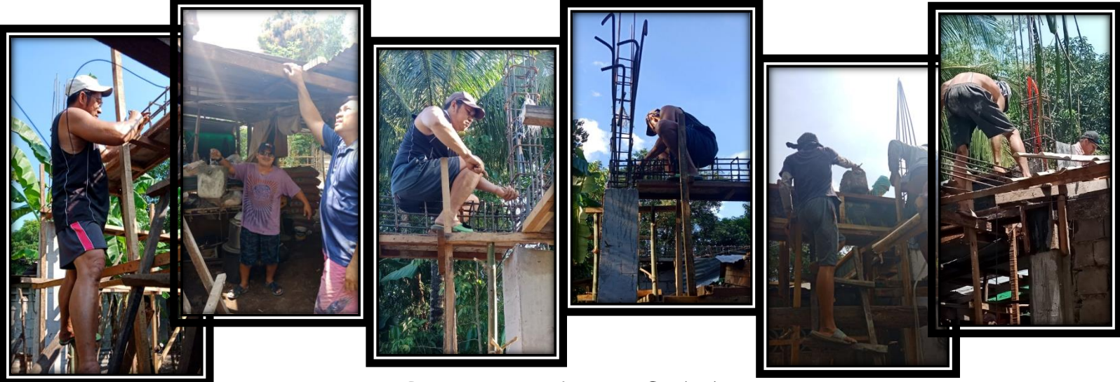
Construction of slab
