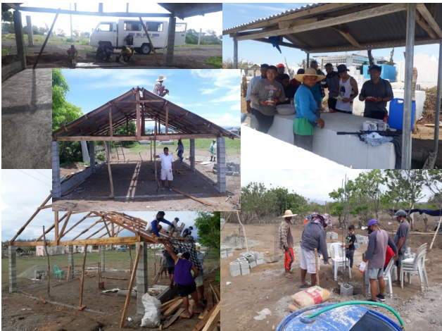
Construction of the Cemetery Chapel
